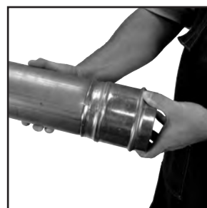
Figure 9: Inspection of final crimp
