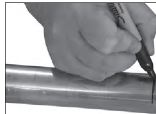
Figure 3 — Marking for Insertion Depth
