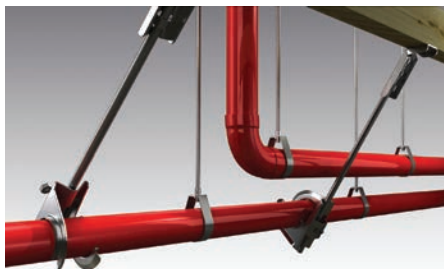
Branch line restraint
